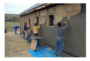
Figure 4.2: Straw Bales coated with plaster
