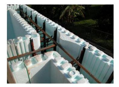
Figure 4.1: Insulated Concrete Form
